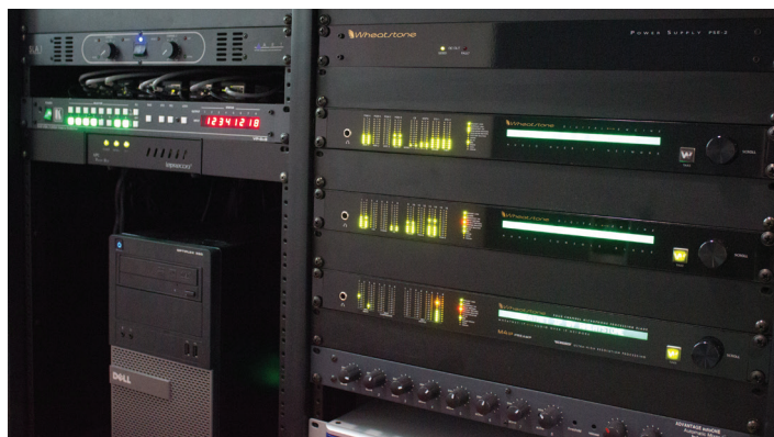
Kramer video matrix switcher (left) for managing studio LCD monitors and Wheatstone Blades (right) for audio and logic routing
