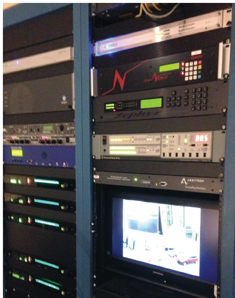
KBEM Equipment racks with Wheatnet blades and Comrex Access
