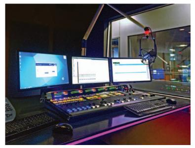
For this market we are using direct wiring to each blade so the only punch blocks will be for tallies and relays. With the standard use of Cat-5e, Cat-6, etc., in AoIP systems, the wiring was easy. All the connectors are RJ-45 on the back of the blades. This allowed us to make use of our networking staff in wiring the new building for audio, which made for a quick install.
