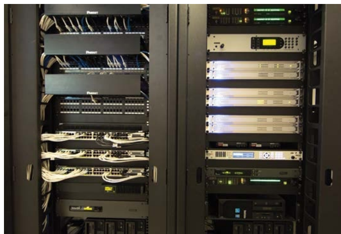
Server Room 407 has two racks dedicated to radio. Middle Atlantic DRK series racks had cable management in the front and back, giving it that finished look.
